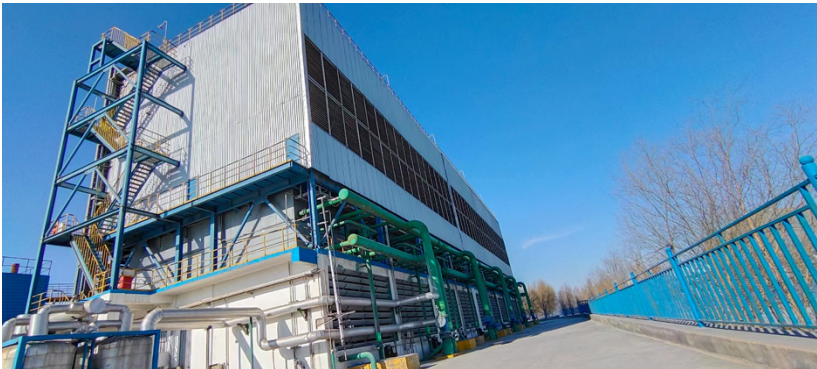
中盐内蒙古化工的密闭循环水冷却塔干湿联合冷却塔
